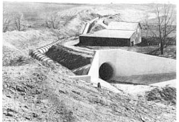
Figure 2-6. Inverted siphon inlet transition and 60-inch-diameter precast concrete pipe. P 499-700-520.
