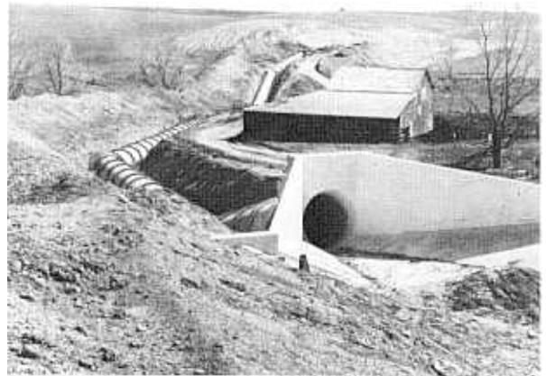
Figure 2-6. Inverted siphon inlet transition and 60-inch-diameter precast concrete pipe. P 499-700-520.
