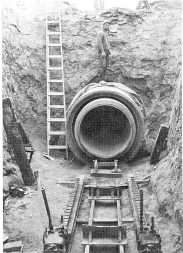
Figure 2-3. Jacking and threading pipe under roadway. P-707-729-2007.
