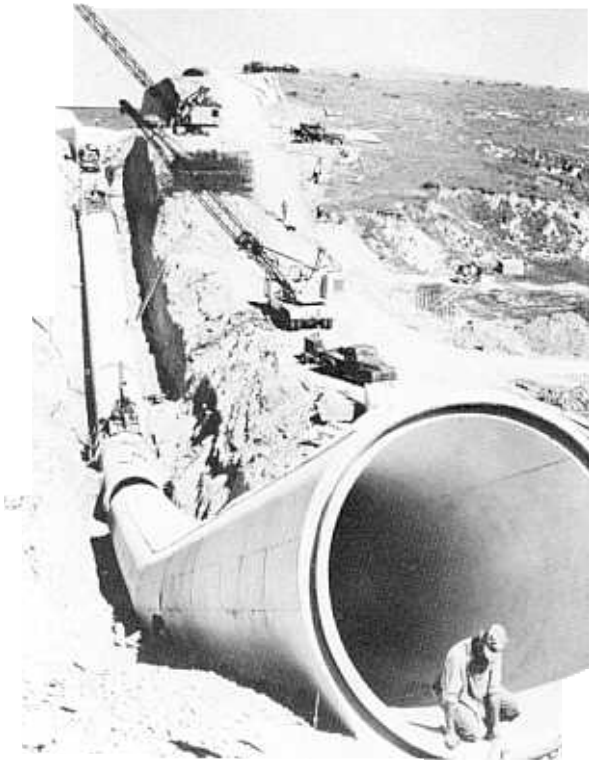
Figure 2-5. Inverted siphon under construction. P-328-701-7259A.
