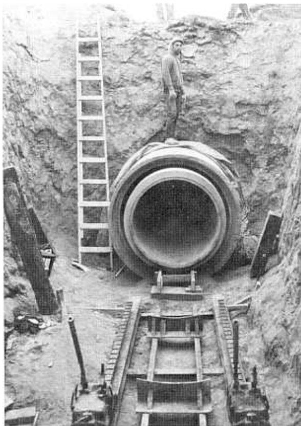
Figure 2-3. Jacking and threading pipe under roadway. P-707-729-2007.
