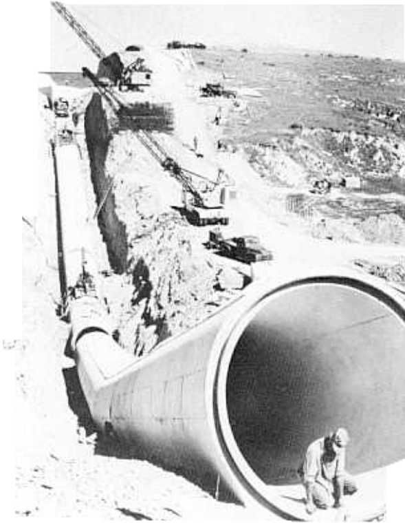
Figure 2-5. Inverted siphon under construction. P-328-701-7259A.
