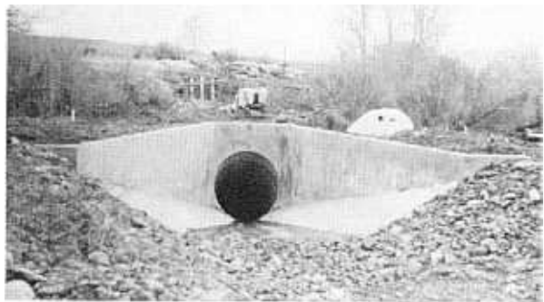
Figure 7-1. Type 1 concrete transition. P33-D-25693
